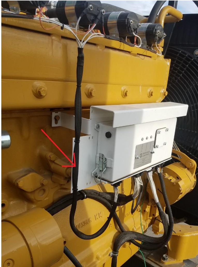
Figure 5. Note ignition harness securely attached to mount bracket to keep it away from other harnesses.
